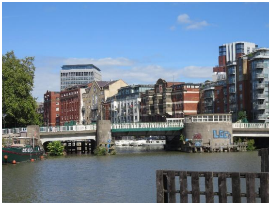
Redcliffe Bascule Bridge from Redcliff Wharf
